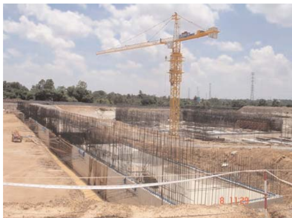
Thu Duc BOO 300,000 m 3 /day Water Treatment Plant being constructed in Ho Chi Minh City
