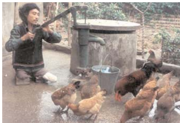
Typical community installed hand pump
