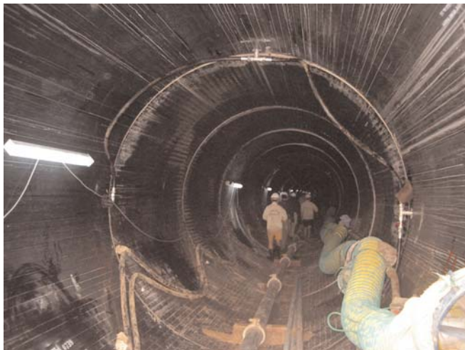
Waste water Interceptor Tunnel under Nhieu Loc Thi Nghe Canal in Ho Chi Minh City
