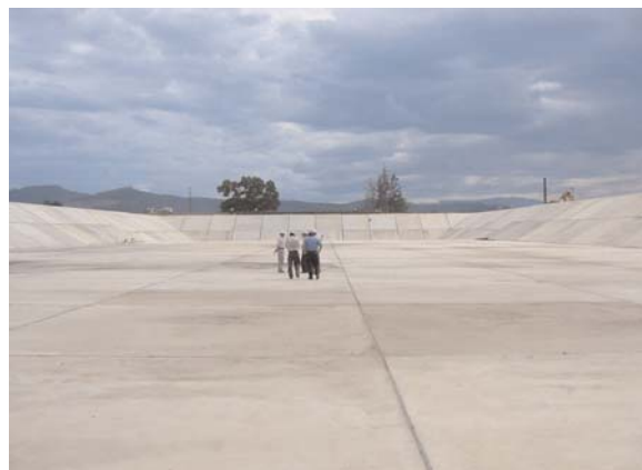
Waste Water Treatment Plant for Danang
