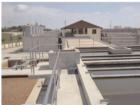
Hanoi Water Business Company's Nam Du Water Treatment Plant
