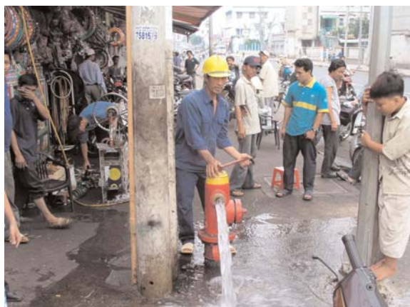
Detecting leaks to reduce non-revenue water
